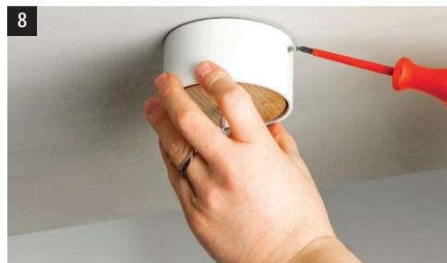
1. Mark the two fixing holes and fit two round-head screws with anchors suitable for the ceiling. Let the screw heads protrude approx. 7 mm.
